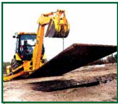
Efficiency's 8x12 Road Plate in use
